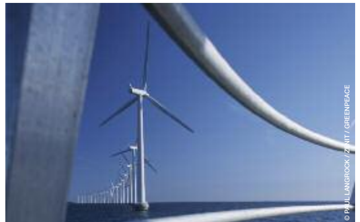
image Off shore windfarm, Middelgrunden, Copenhagen, Denmark.
